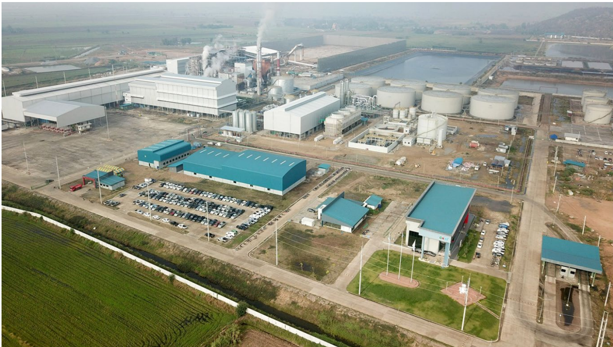
Figure 3.34. Bioethanol Factory in Thailand
