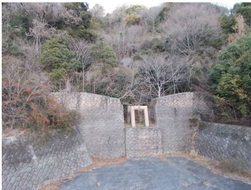
Figure 5.9. Sabo Dam in Rokko Area
